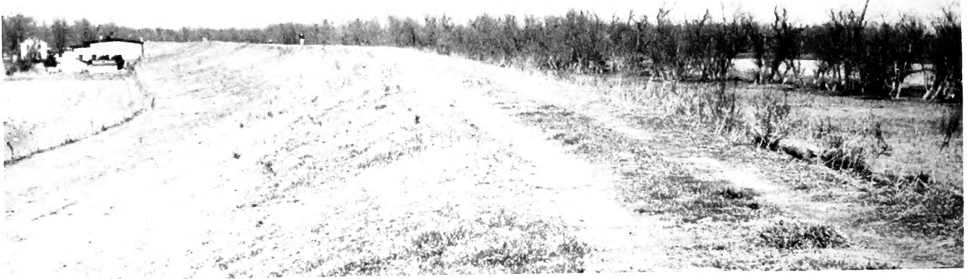
Fig. 1.--Typical Illinois River levee. Part of the Illinois River is visible at right and margin of a drained lake basin, planted to corn, at left. In background at left is pumping station.
